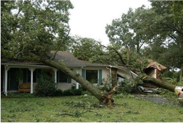
Figure 3-9 Home Damaged During Windstorm
