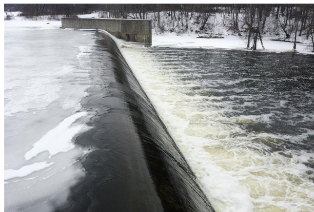
Figure 3-14 Goshen Pond Dam (James Buck)
