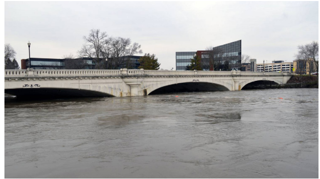
Figure 2-11: 2018 Flooding in South Bend
